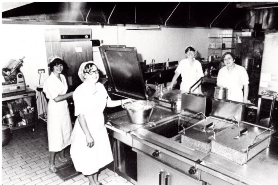
Part of the kitchen area which caters for 1000 staff.
